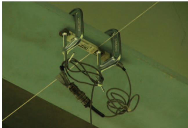
Fig. 1. Reusable strain transducer mounted to the lower flange of a beam
