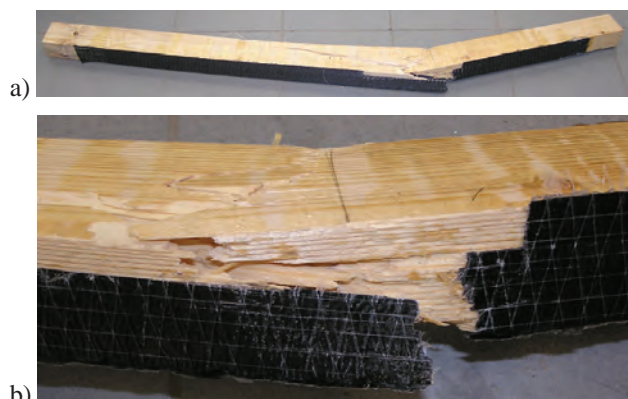
Fig. 11. View of the destroyed beam reinforced with composite sheet from carbon fibers S&P C-Sheet 240/400 (two – layer reinforcement), a) the whole element, b) closer view
