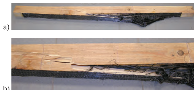
Fig. 10. View of the destroyed beam reinforced with composite sheet from carbon fibers S&P C-Sheet 240/400 (one – layer reinforcement), a) the whole element, b) closer view
