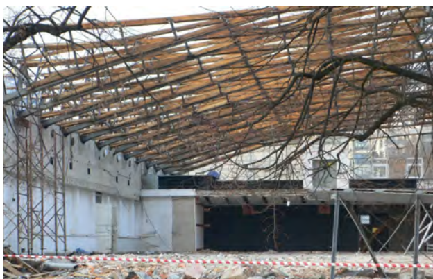
Photo 10. The supermarket during demolition (source: culture.pl)
