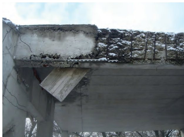
Fig. 6. Part of monolithic lintel with missing cover
