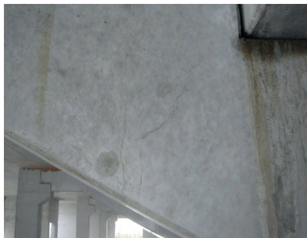
Fig. 7. Cracks on the tribune beam on the 2nd floor
