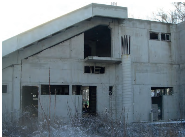
Fig. 5. Incorrectly static distribution of holes in the load-bearing wall
