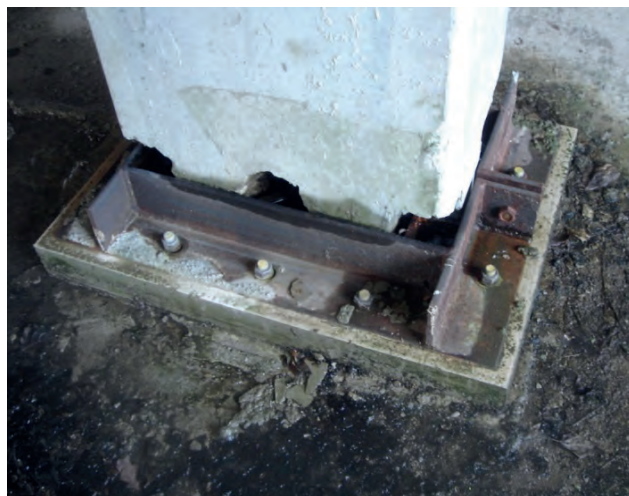
Fig. 8. Detail of incorrect anchoring of columns
