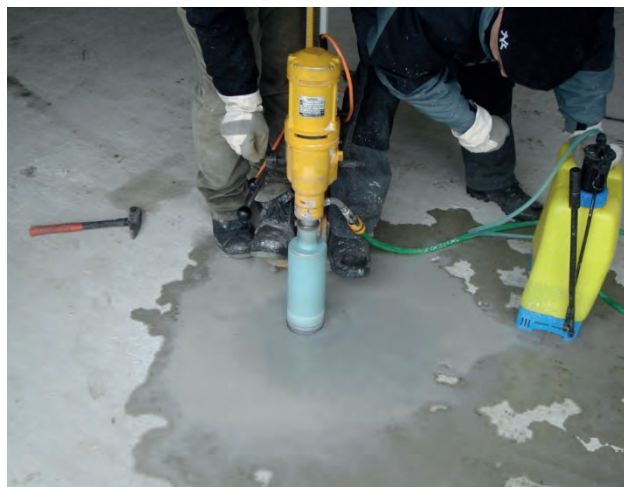
Fig. 4. Core borehole in the slab (2nd floor)
