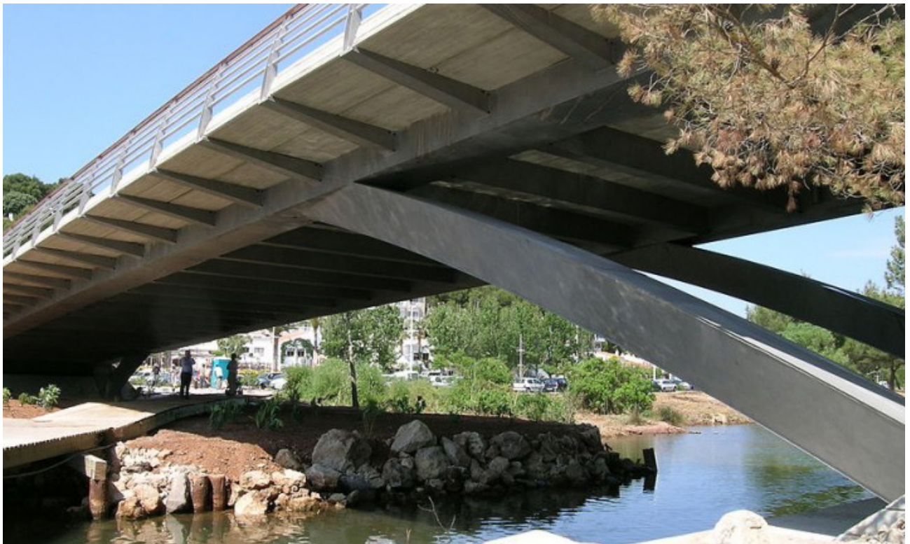
Fig. 2. Cala Galdana Bridge on Menorca (Spain) [6]
