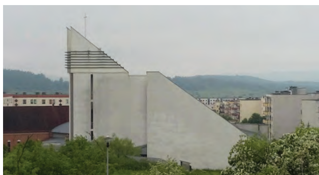
Fig. 2. Church of Bł. Jerzego Matulewicza – general view of the building structure, Kielce – Oś. Ślichowice, 1993-2003-2005, designers expansion of the church Piotr Bielański i Krzysztof Filuś, photo by author, 2015
