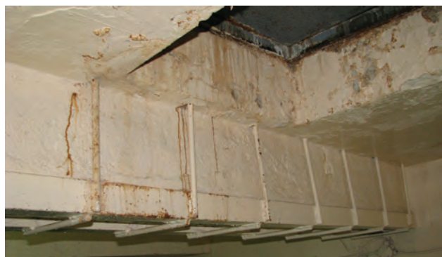
Fig. 2. View of corrosion of the floor and floor beams at the level of +4.20 in part B
