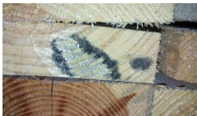
Fig. 8. Blue stain in construction and structural sawn timber and round timber
