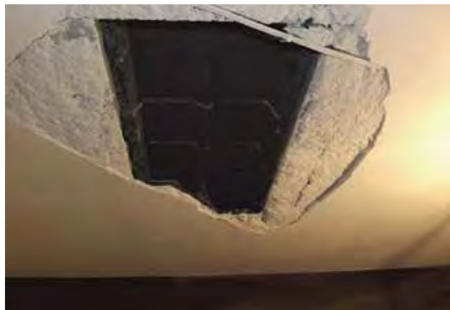
Fig. 1. Bottom section of the filler block fallen away
