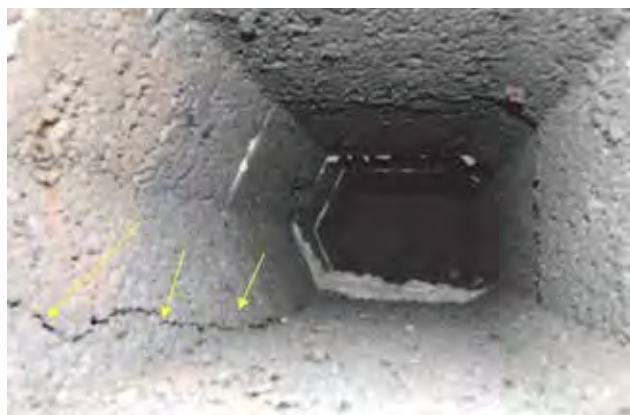
Fig. 4. Floor filler blocks with visible cracks indicative of disintegration of their bottom faces
