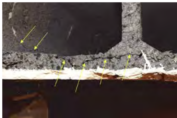
Fig. 4. Floor filler blocks with visible cracks indicative of disintegration of their bottom faces
