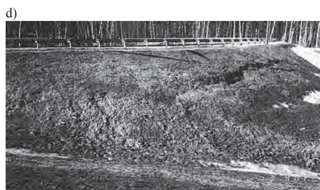
Fig. 1. Local deformations of subgrade embankment: a) road in Alaska [4]; b) Qinghai - Tibet railroads [3]; c) Russia – road «Yamal» [1]; d) Russia – road «Don» 104 km [1]
