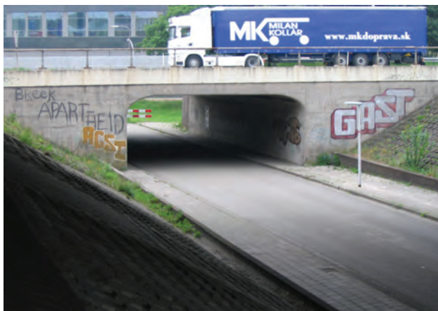
Fig. 3. Solid slab bridge deck
