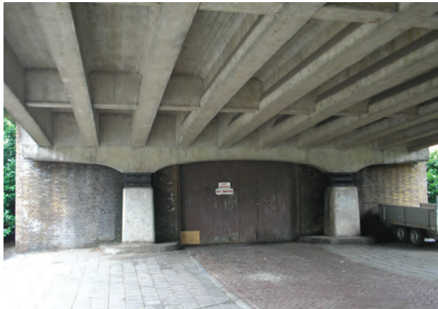
Fig. 2. T-beam bridge deck
