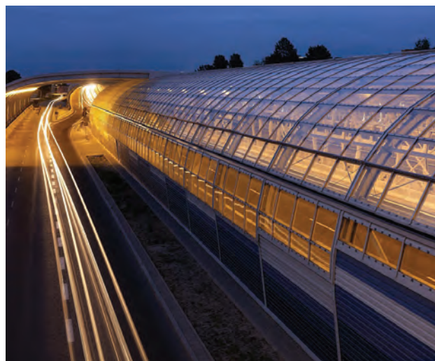
Fig. 7. External view of the half-tunnel noise barriers [14]
