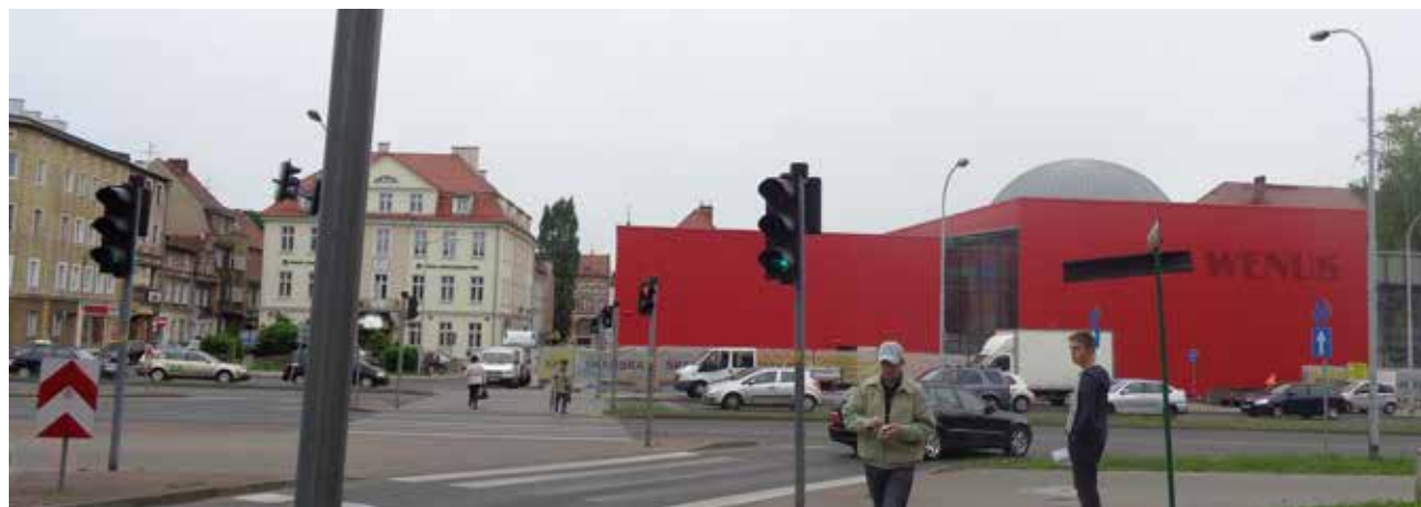
Fig. 4. View of the Town Hall from the side of Gen. W. Sikorskiego street in Zielona Góra. Year 2015. Source: author
