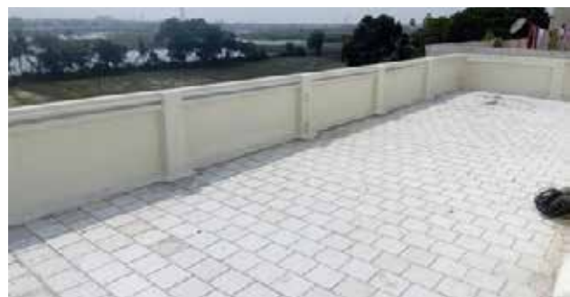
Fig. 4. Roof with mounted cool tiles [17]
