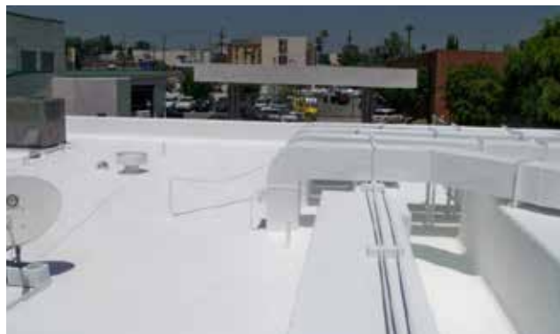
Fig. 3. Roof painted with cool paint [17]
