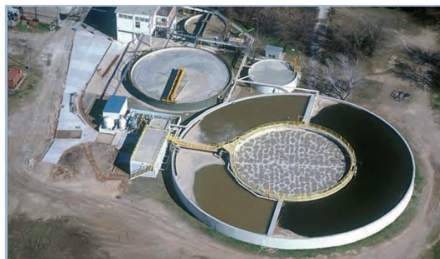
Fig. 4. Unitank configuration in the round module. Rousselot, Argentina [9]
