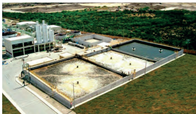
Fig. 3. Basic Unitank configuration in the square module. Pemex, Mexico, oil company [9]
