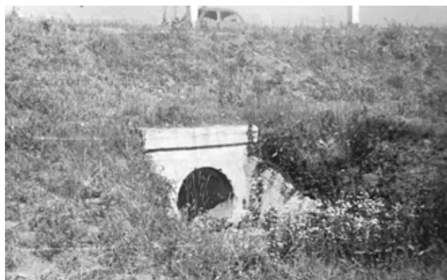
Fig. 1. Road-bed and pipe culvert at km 122+629 of Moscow-Voronezh motorway. Pipe diameter 0.75 m
