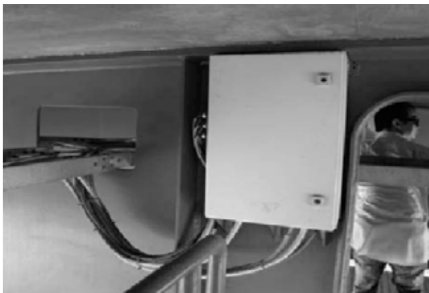
Fig. 7. Temperature sensor install on main girder of Rao II Bridge during inspection
