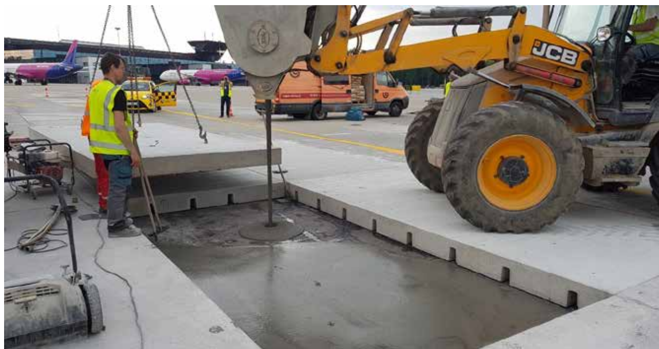
Fig. 6. Installation of a prefabricated concrete slab
