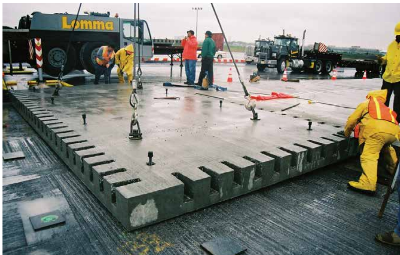
Fig. 1. Prefabricated PCP concrete slab used at La Guardia International airport in New York [2]
