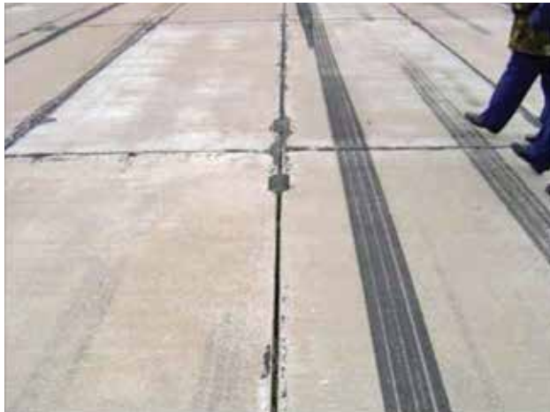
Fig. 2. Prefabricated slabs used in the USSR (on the left airport slabs, on the right – the technique of connecting staples) [1]
