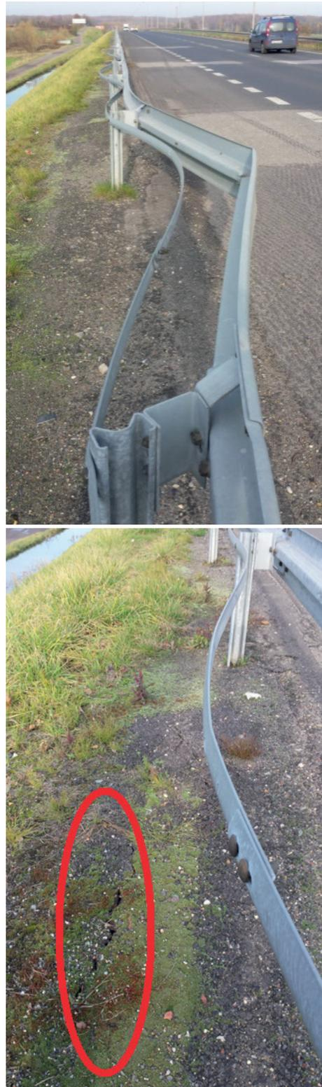
Fig. 16. Longitudinal crack in the crown of the embankment along with the deformed road barrier
