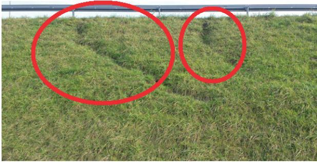
Fig. 17. Vertical slots in the embankment corpus
