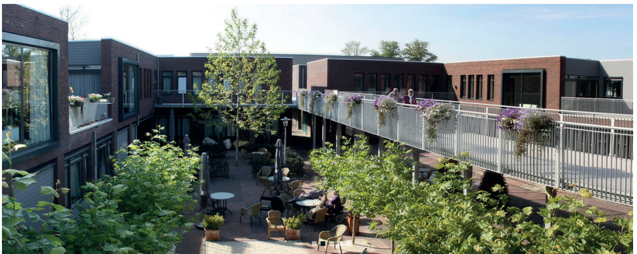
Fig. 4. Hogeweyk housing estate in the Netherlands
