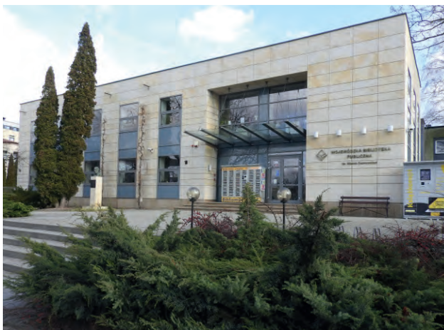
Fig. 9. Entrance to the Public Library from the front side
