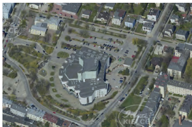
Fig. 2. View of the KCC building
