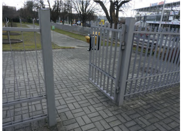
Fig. 12. Passage through a gate to a wheelchair-accessible area
