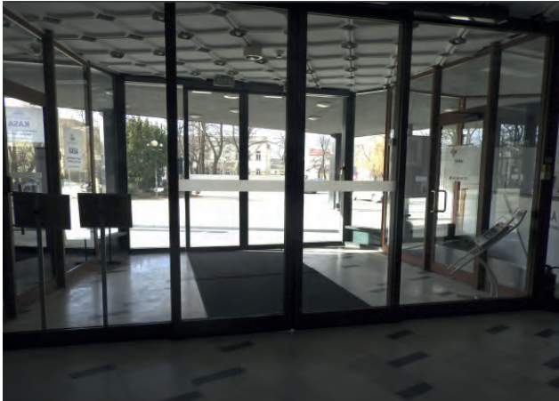
Fig. 5. Main entrance area with glazing markings
