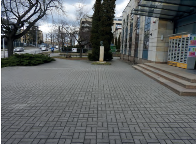
Fig. 11. Pavement zone on the front side
