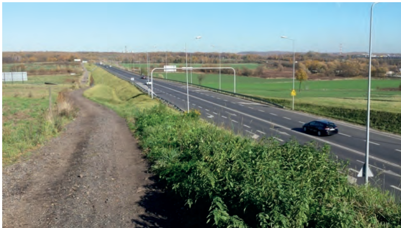
Fig. 5. Northern bypass of the Upper Silesia Agglomeration in Bytom, a section of the route that runs on an embankment visible in the distance, October 2018
