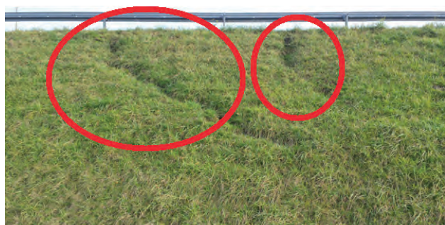
Fig. 17. Vertical slots in the embankment corpus
