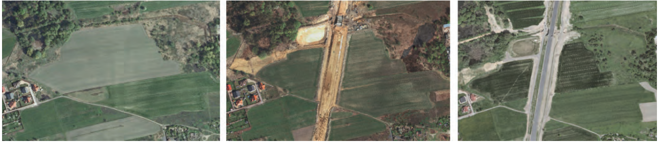
Fig. 6. Orthophotos from the years: 2009, 2011 and 2012 – completion of embankment construction source: http://geoportal.gov.pl
