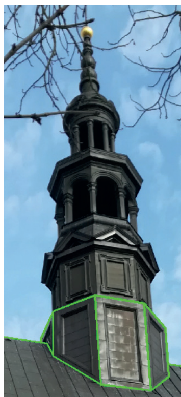
Fig. 4. Tower of the Cathedral Basilica of the Assumption of the Blessed Virgin Mary in Kielce. Interpenetration line of the tower with the roof (photo taken for the analysis of the problem 1). Next: a 3D model of the connection between the tower and the roof used for the geometric analysis of the structure Several AutoCAD visualization options: 3D wireframe, conceptual, 3D hidden, sketchy
