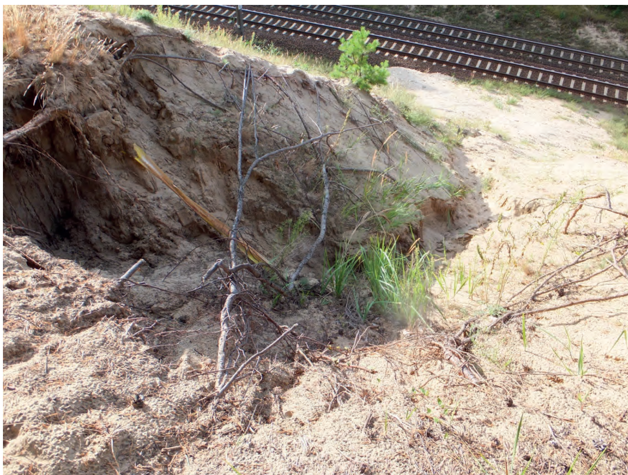
Phot. 1. Erosive funnel with washed-out fine sandy material. Photo by Tomasz Sobkowiak
