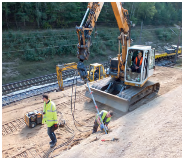
Phot. 2. Installation of CHANCE non-injection nails. Photo by Tomasz Sobkowiak
