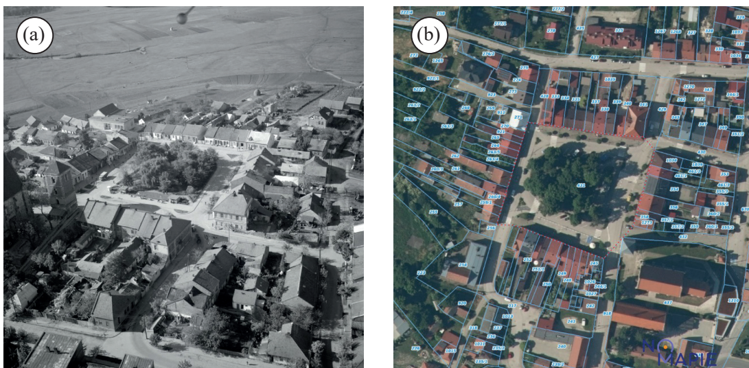
Fig. 5. Wiślica – Market Square: (a) Condition in 1967 [Source: [4]]; (b) Current condition. Aerial photograph taken on 27.05.2024 [Archival aerial photograph report, retrieved: 07.05.2026]
