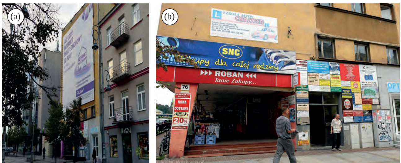
Fig. 10. Example illustrating the mechanism of advertising chaos – Kielce, 76 Sienkiewicza Street; upper floors fully covered by a large-format banner (a) [32], excessive concentration of advertisements at ground level (b) [33]
