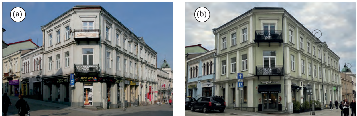
Fig. 15. Comparison of the facade at 17 Sienkiewicza Street before (a) [36] and after (b) the implementation of the landscape resolution [Source: J. Lech]
