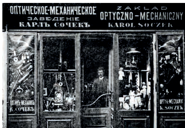
Fig. 3. Shopfront of Karol Soczek’s Optical and Mechanical Workshop in Kielce – example of late 19th-century commercial signage integrated with the architectural composition of the facade [25]
