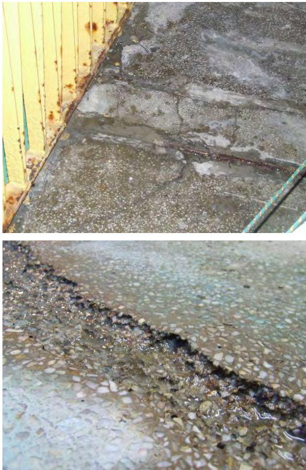
Fig. 1 Corroded area of the concrete floor and exposed rebar in an indoor swimming pool
