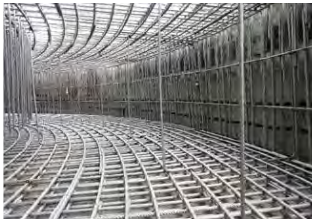
Fig. 7. Reinforcement made of stainless steel [14]
