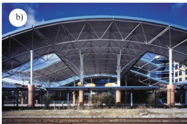
Fig. 2. Roofing of Lynx Central Station in Orlando, Florida: a) general view; b) view of the structure [17]
